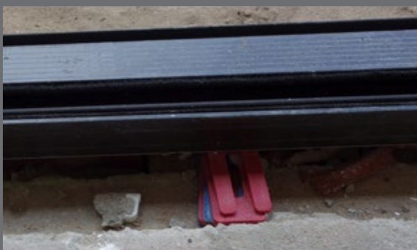
✓ SILL PACKED CORRECTLY
